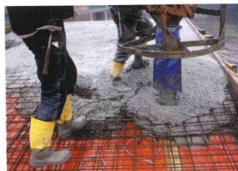
In-situ reinforced concrete being poured
